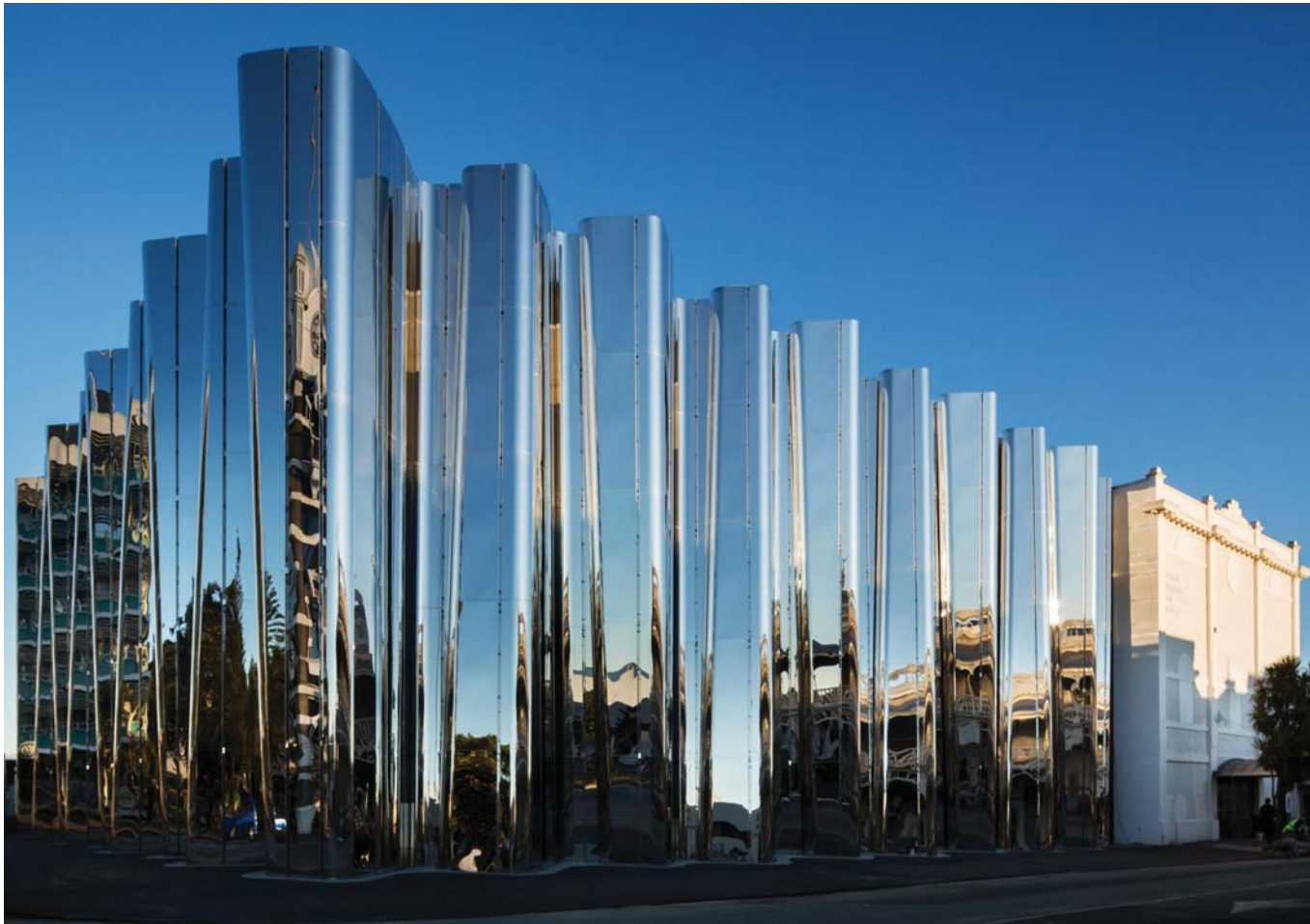
Photos by Patrick Reynolds, courtesy of Patterson Associates
