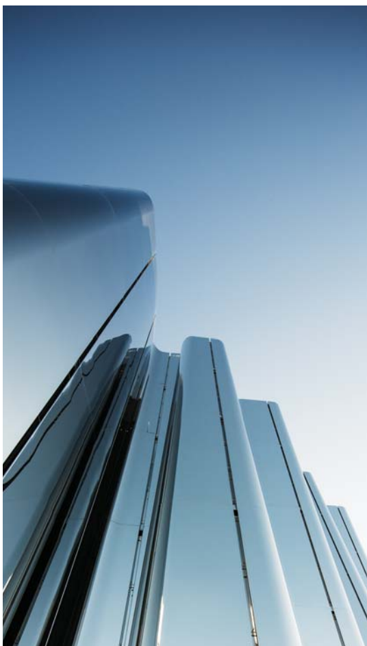
Type 316 stainless steel was polished to the highest possible level, to ensure maximum corrosion resistance and achieve mirror-like appearance.
